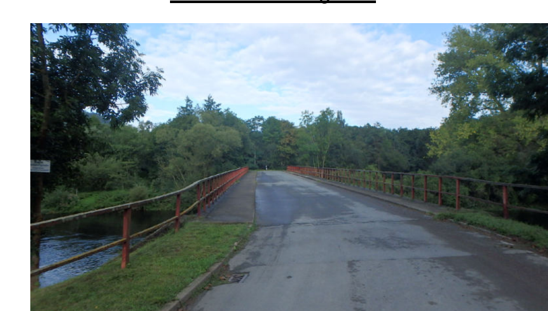
Blick in Richtung B85
